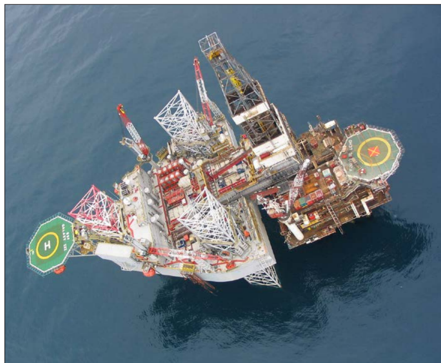
North sea oil rig
